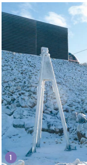
TRIPOD GROUND ANCHRAGES PYRAMID
