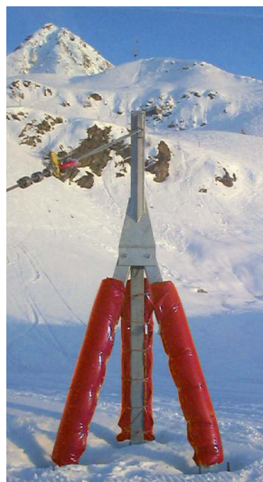
TRIPOD GROUND ANCHRAGES PLATE
